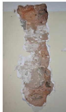
Fig. 21 Detail of the materials granulometry of a wall
