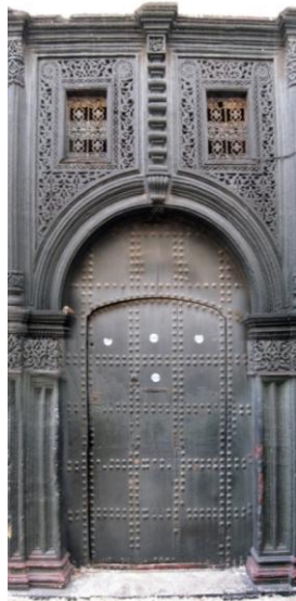
Fig.6 View of the main door ( bab el Dar )
