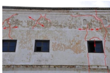
Fig. 23 Detail of features on the main elevation
