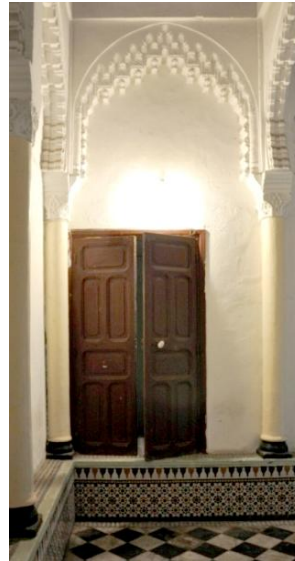
Fig.7 View of the satwan with the dukkan
