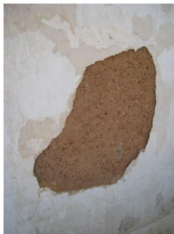
Fig. 20 Detail of the wall in Pisé of the Dar Dgi'ra
