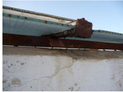
Fig. 29 Detail of the iron-glass roof
