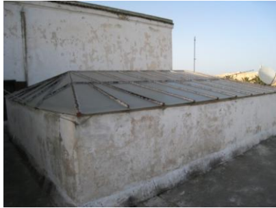
Fig. 28 View of the iron-glass roof from the terrace
